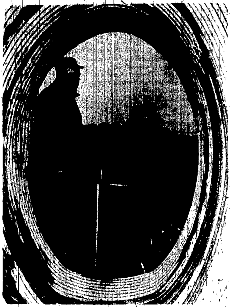
BEEF CATTLE on the Ray Agler farm northwest of Wayne are now using this underpass culvert to cross from one field to the other. Agler is shown just outside the culvert, the first of its type installed under a Wayne County road.
